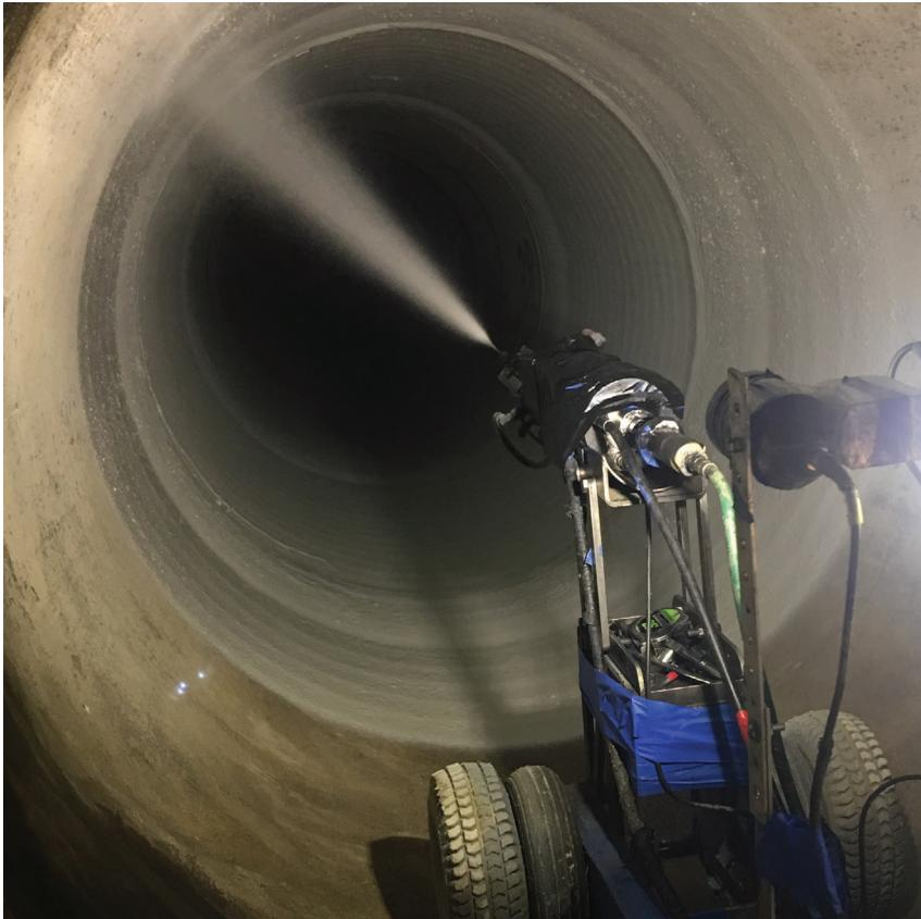
**Nukote Aegis®** Liners differ depending on the effluent type, abuse levels, abrasion, ground movement, substrate condition and other design variables. The application processes are similar, the liner formulation utilized is variable.
