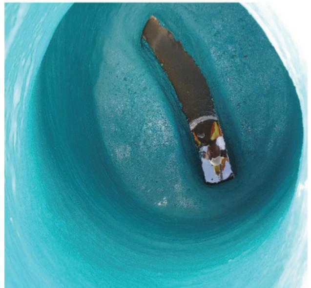
**Nukote Aegis®** Liners are installed using high pressure, heated, plural component proportioning equipment. The applications are performed either manually or utilizing **Nukote 360Ringtech® Robotics**.
